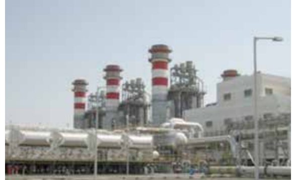
Suhar desalination plant - Sultanate of Oman
